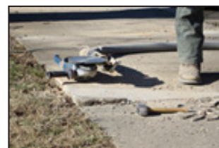
Sidewalk grinding
