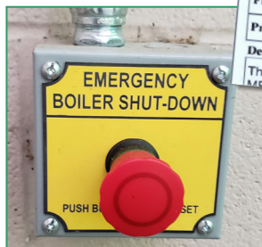
Central Plant emergency shut off at each exit
