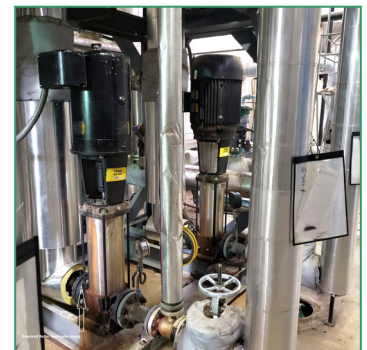
Repaired feed water pumps
