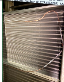
Coil replacement Rec Center
