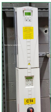
New cooling tower drive
