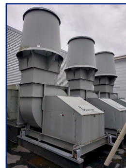
Air Vents for 160 Fume Hoods at New Science Building
