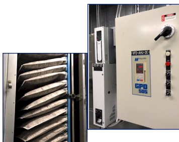
Variable Frequency Drive at AHU and Filter Bank
