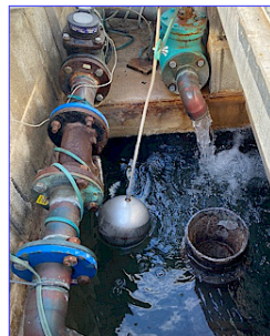
Cooling Tower N & S Float Replacement
