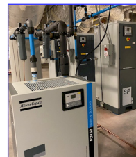
New Air Compressor System- New Science Building
