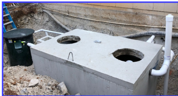
Starbucks – New Grease Trap Installation
