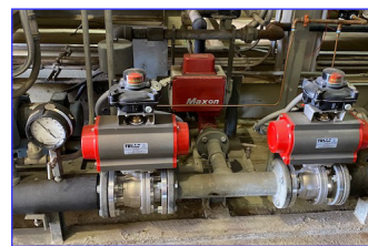
Heat Recovery Boiler Gas Valves
