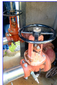
Valve Replacements
