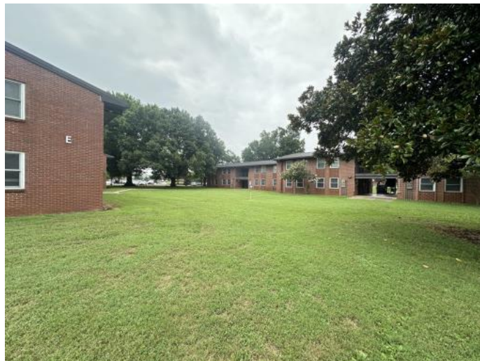
Photo 10 Site View Facing Northeast near B-3
