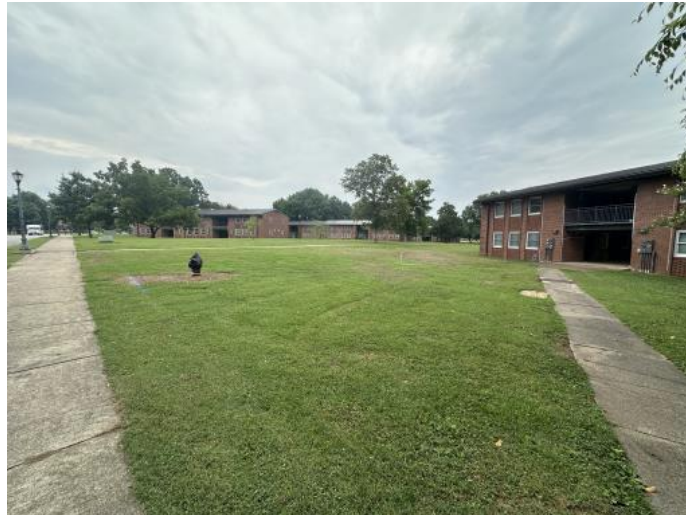
Photo 9 Site View Facing Northeast near B-5
